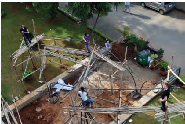
Figure 9.7 Placement of bent pipe edge curves
