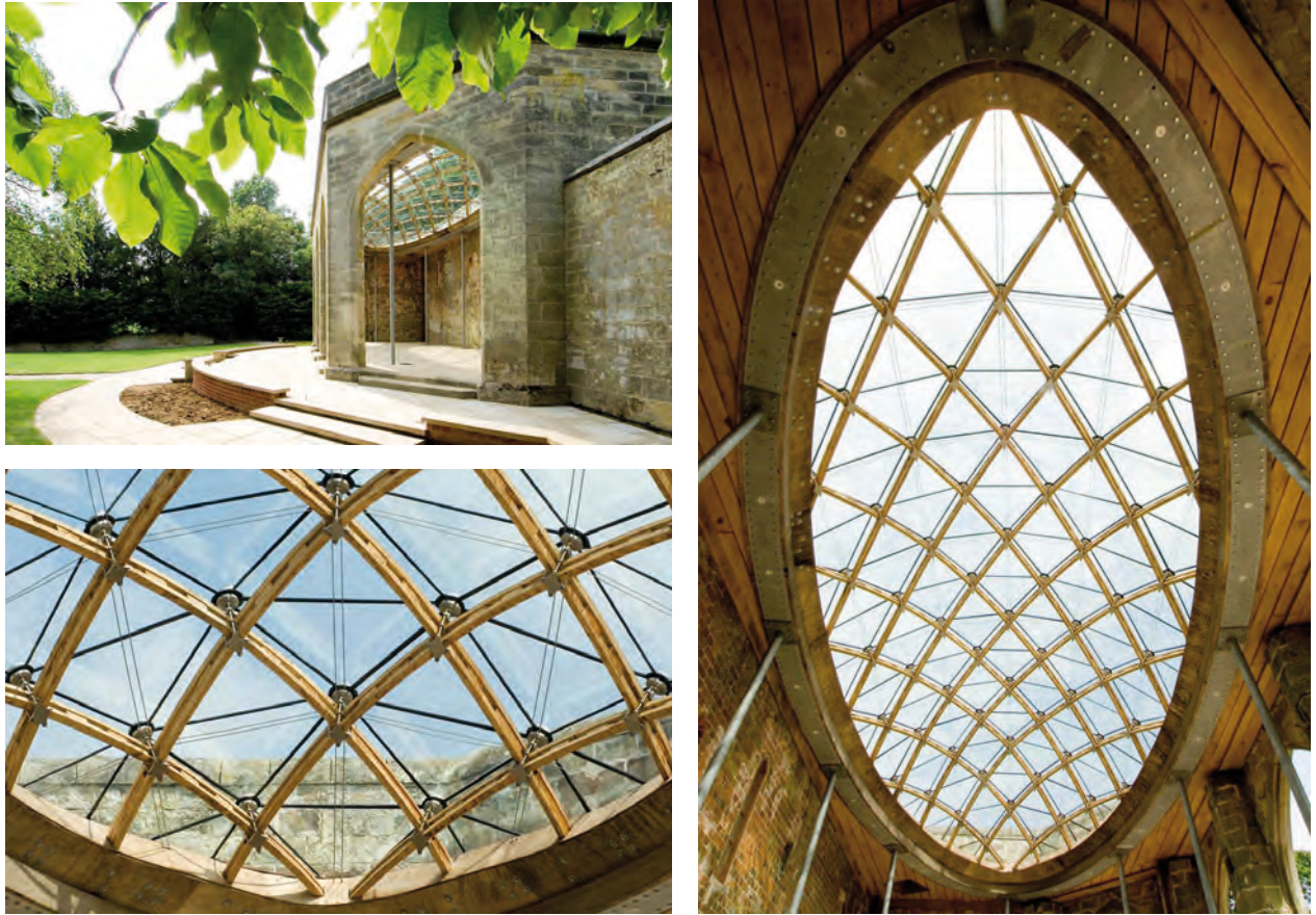
Figure 8.4 The double-layer gridshell with external bracing of the Chiddingstone Orangery in Kent, UK, 2007
