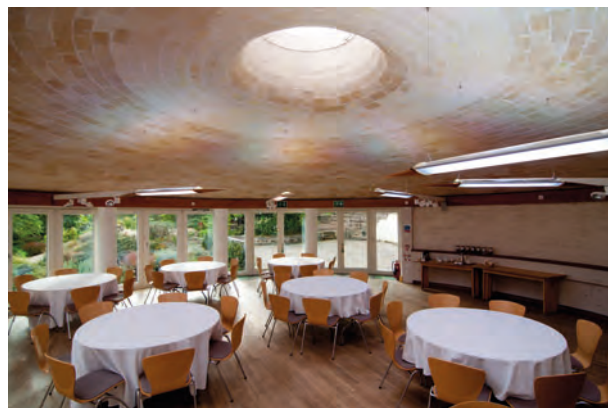
Figure 1.4 (top) Conical shell by Rafael Guastavino, Sr., Bristol County Courthouse, Taunton, MA, 1891, (middle) shallow spherical dome, Bronx Zoo Elephant House by Rafael Guastavino, Jr., New York City, NY, 1909, and (bottom) shallow spherical shell with upturned oculus, Pines Calyx by Helionix Designs, Dover, 2007.
