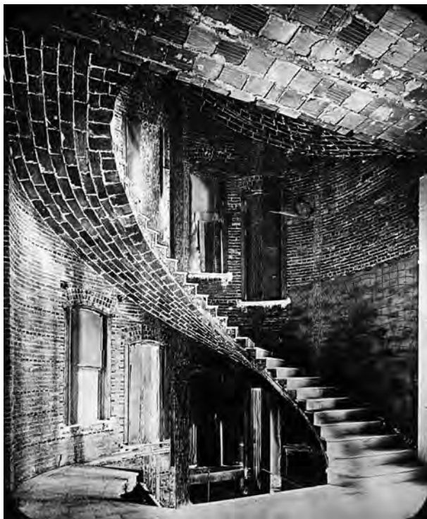
Figure 1.6 Guastavino thin-tile helicoidal stairway at the Union League Club, New York City, NY, 1901, and the force equilibria of (a) a dome with a circular oculus, (b) a circular flat vault with an oculus, and (c) a spiral stair can be explained with (d) the same force pattern topology, with radial arches and meridional hoops. The horizontal thrusts are balanced in the same manner, as visualized in (e) their shared reciprocal force diagram (see Chapter 7).
