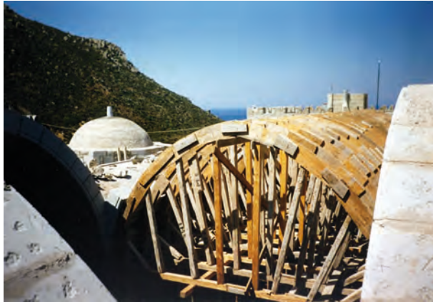
Figure 2.3 (top) One of many vernacular, curved structures in the Cycladic islands, and (bottom) a typical formwork for a vault
