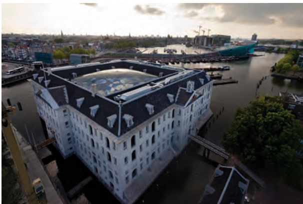
Figure 2.6 The Dutch National Maritime Museum as seen from outside revealing the faceted gridshell
