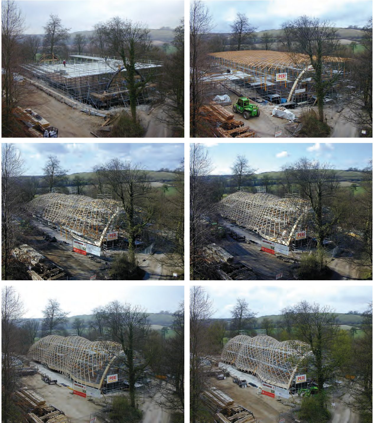
Figure 8.13 The lowering process for the Downland gridshell
