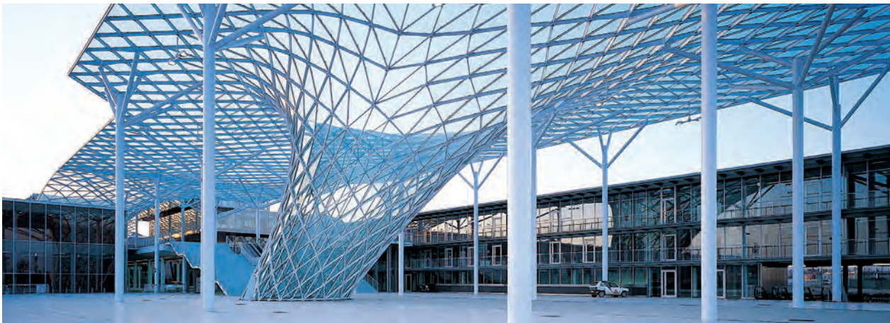
Figure 15.1 Roof of the New Trade Fair, Rho-Pero, Milan, Italy, 2002–2005, by Massimiliano and Doriana Fuksas architects, with a grid mapping onto a complex surface
