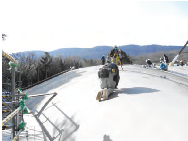
Figure 21.15 Shape measurement of the formwork
