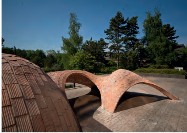
Figure 7.1 Tile vault prototype at ETH Zurich, Switzerland, 2011
