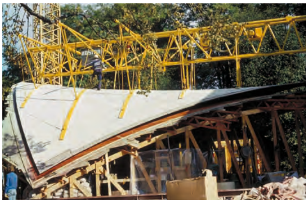
Figure 0.1 Bundestgartenschau Pavilion, with a 12mm fibre reinforced concrete shell, Stuttgart, 1977
