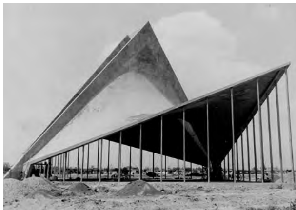
Figure 0.3 Hypar shell with direct edge beam supports for the Church of San José Obrero by Félix Candela, Monterey, 1959
