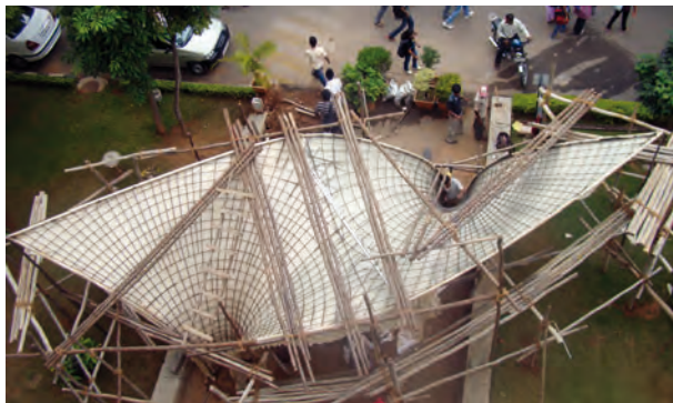
Figure 9.10 On-site fabric guidework with rebar in place
