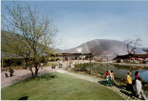
Figure 19.1 The gridshells for the Mannheim Multihalle
