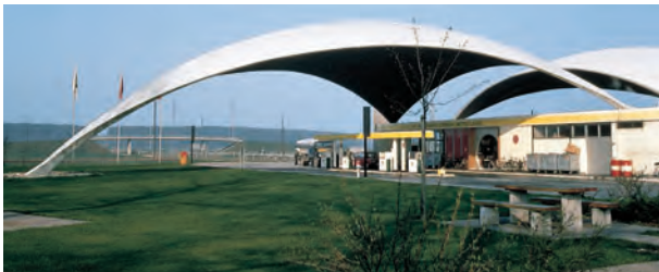
Figure 20.11 BP Service Station, Deitingen, 1968
