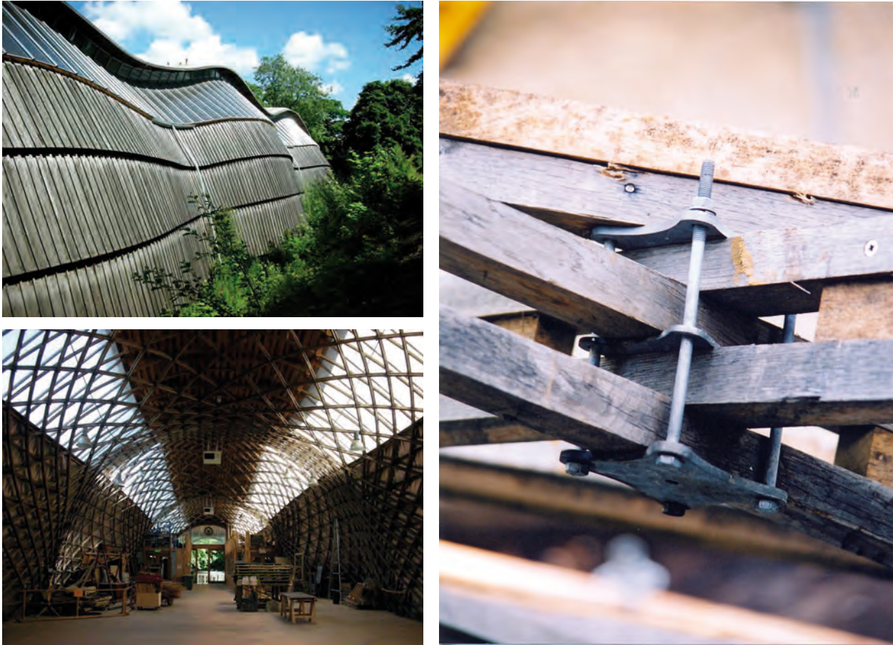
Figure 8.12: Downland gridshell, Chichester, UK, 2002, with (top left) western red cedar cladding, (bottom left) housing a workshop and (right) detail of connectors
