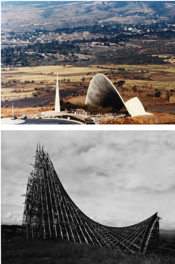
Figure 20.5 (top) Chapel Lomas de Cuernavaca, 1958, and (bottom) falsework used during construction showing straight wood formwork
