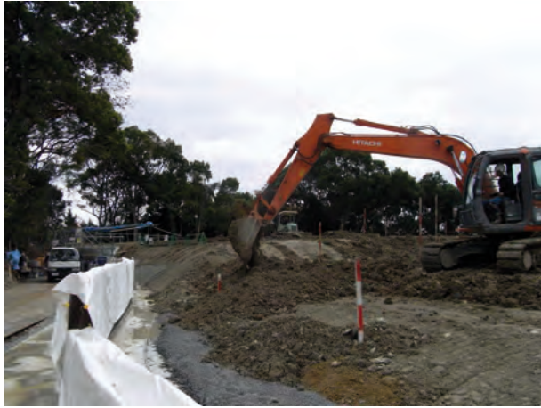
Figure 21.14 Formation of the earth-filled formwork
